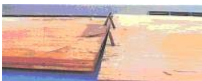
inadequate nailing
