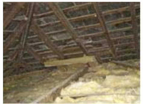
roof space with chimney breast removed
